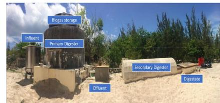
Figure 5: Anaerobic digester at Center for Sustainable Development
