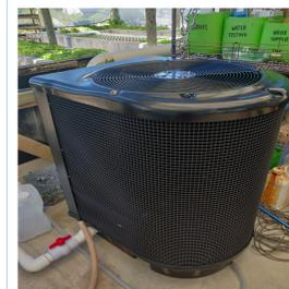
**Figure 3:** The chiller keeps the water temperature consistently at 26°C.
