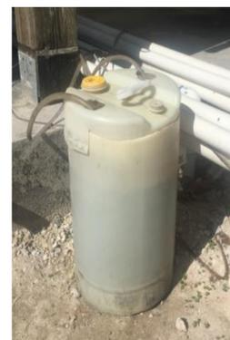
Figure 6: 15 gallon plastic mineralization vessel
