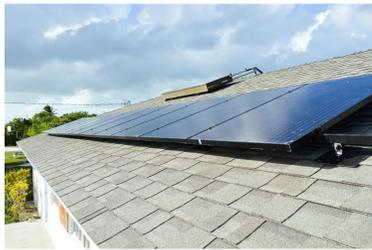
3.6 kW solar PV array installed on DCMS.
